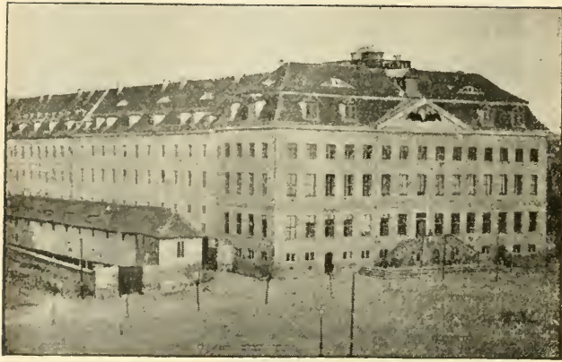
FRANKE ORPHAN HOUSE, Halle, Germany.
